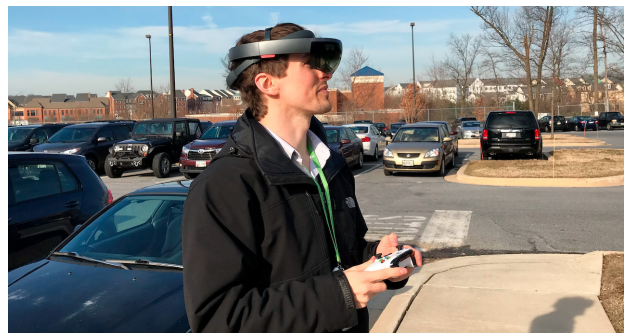
Figure 2. Stephen Bailey demonstrating the use of the HoloLens and controller on the construction site. The existing 3-D model was imported into Unity to create an application for the HoloLens that enabled the wearer to walk around the B201 construction site and see the shell of the building in its expected place.
