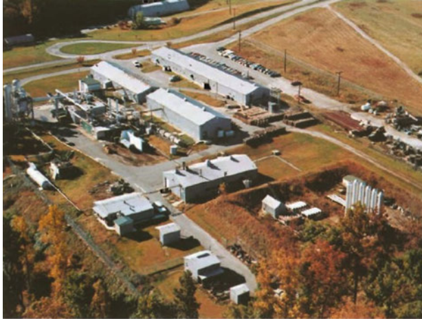
Figure 4. PRL complex of multiple buildings and innovative facilities to support hypersonic testing.
