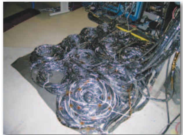
Figure 9. Cabling for one spacecraft outside the GSFC thermal vacuum test chamber.
