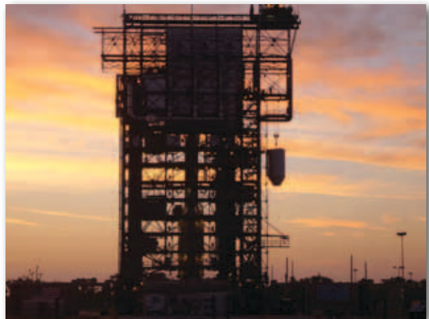
Figure 13. Lifting both STEREO observatories to the top of the launch tower.
