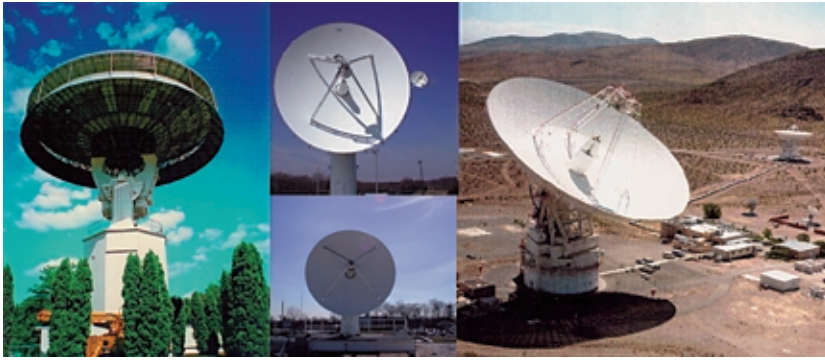
Figure 6. Collage of the APL 60-ft (left), 10-m (center top), 5-m (center bottom), and Deep Space Network 34-m (right) antennas. All are currently supporting APL mission operations. Not shown is an AFSCN network antenna, which is also being used to support MSX.
