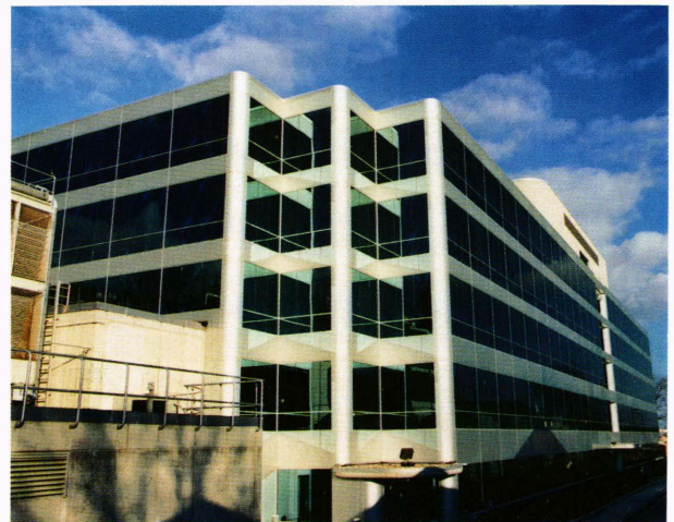
Figure 3. The Steven Muller Center for Advanced Technology.
