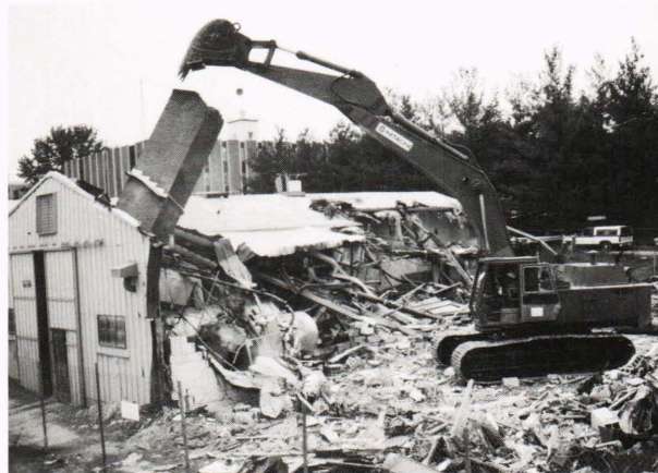
Figure 2. Demolition of old Building 13 circa June 1987.
