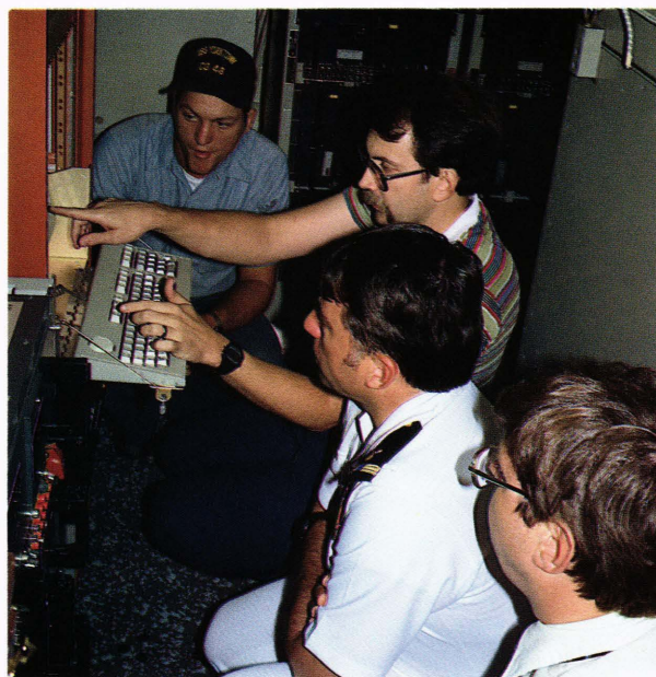
Aboard USS Yorktown , Ken Plantz, APL, demonstrates to CWO Dan Pinto, Combat Systems Test Officer, a portable data processing unit that the APL team had just installed in the Yorktown Computer Central facility. Watching are FCM-2 Robert Turner, USS Mahan , and Bill Mehlman, APL.
