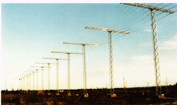
Figure 4 —View of the original antenna array from the front, northwest corner. The shed containing the phasing matrix, array select logic, and power supplies is located at the center of the array.
