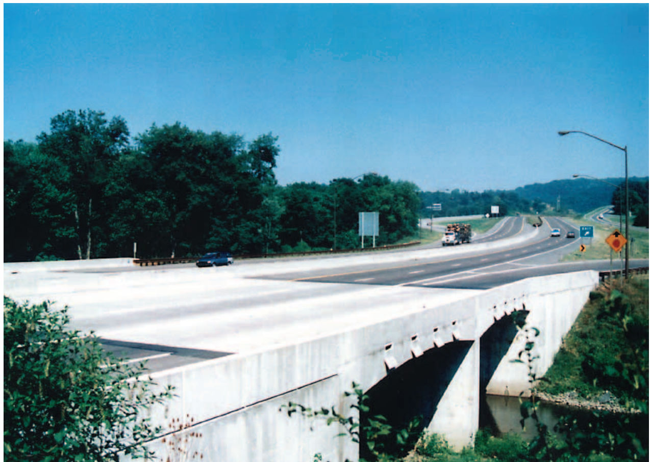
Figure 4. Picture of the 93 × 133 ft concrete bridge, which is CP protected. The CP current on this bridge was mapped using magnetic sensors over a period of 4 h.
