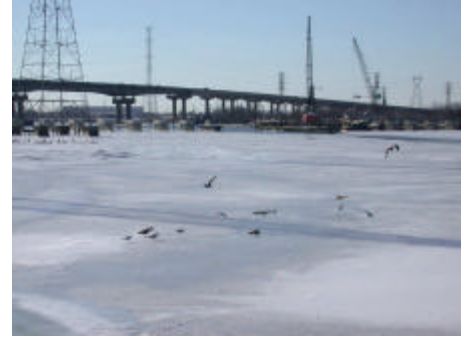
I-495 BRIDGE OVER CHRISTINA RIVER, WILMINGTON, DELAWARE..
