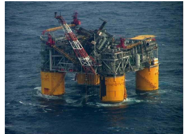
Gulf Rig Destroyed by Katrina
